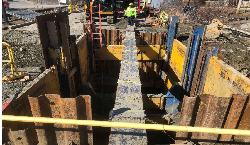
Slide Rail Support of Excavation
